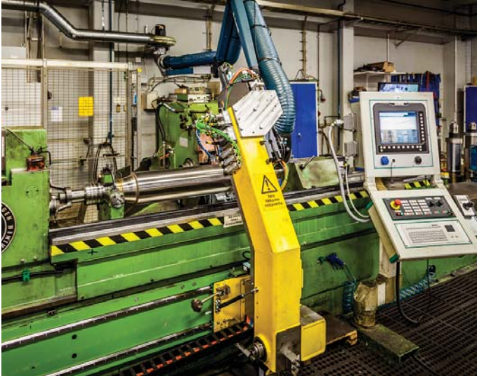
Herkules work roll grinder, modernized in 2015
